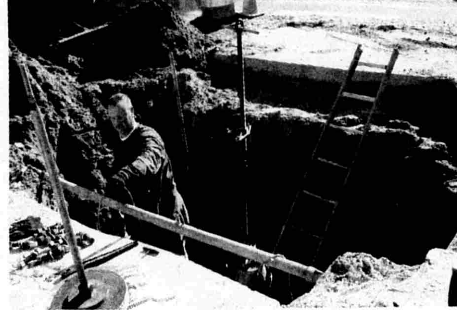
Eric Wsolek of Watertap Inc. works on a 12" main line stop as part of the utilities relocation project. Michigan Department of Transportation along with the city are readying for the upcoming downtown bridge replacement project - slated for spring start.
