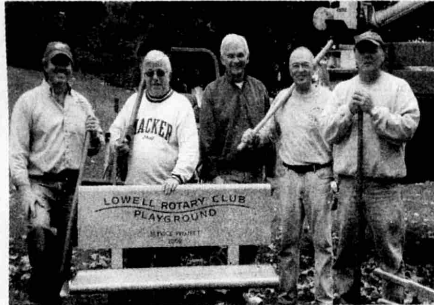
It was another work day at Richards Park on Oct. 20 as volunteers installed a granite bench. The bench was installed inscribed on the back with the names of some of the major donors. On the front are the words "Lowell Rotary Club Playground Service Project 2009." Rotarians working on the playground are pictured, left to right: Jeff Wilterink, Richard Bryan, John Gruzenza, Jim White and John Sterly.
