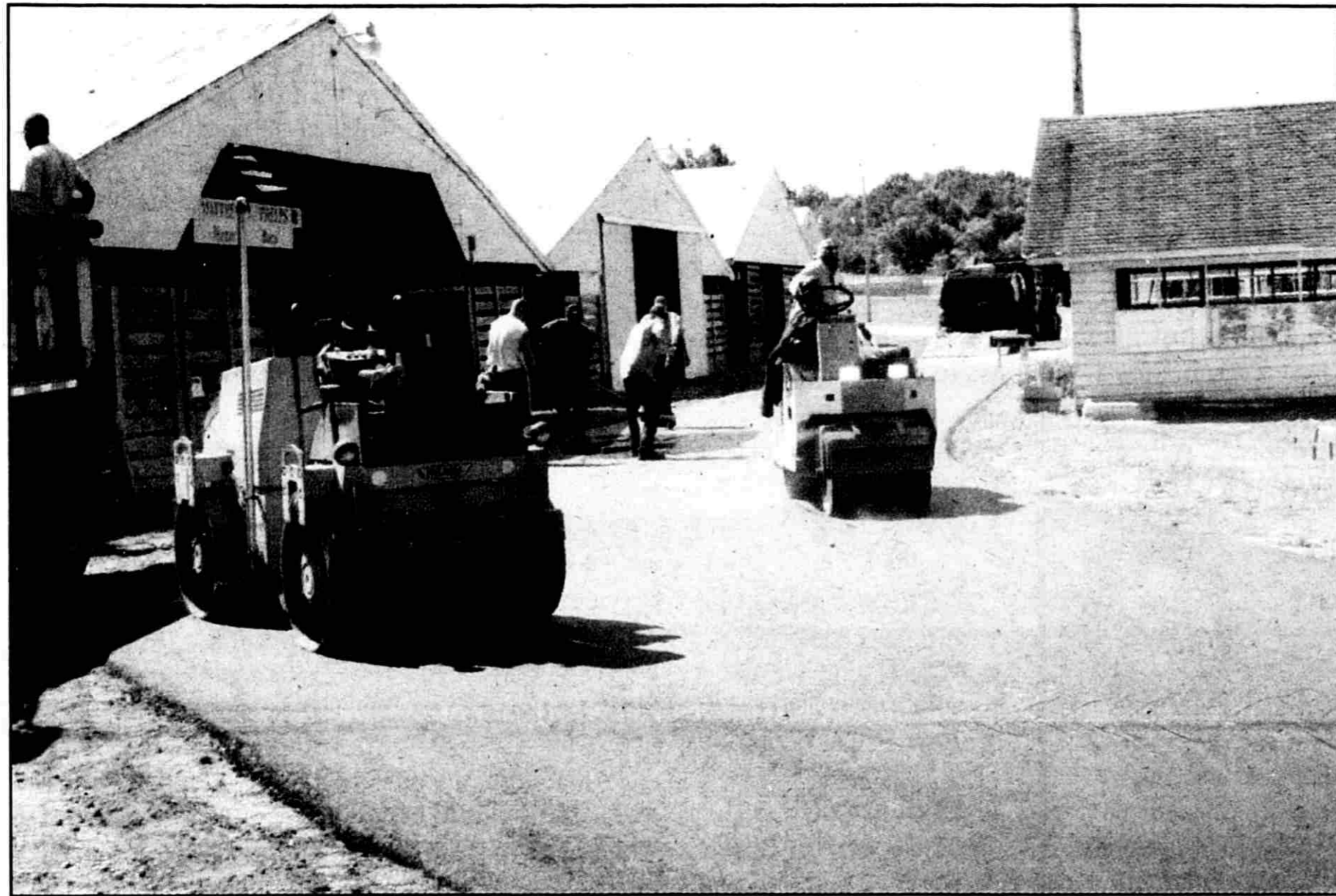
Howard Russell of Superior Asphalt works on blacktopping the area between the food concessions and the barns.
