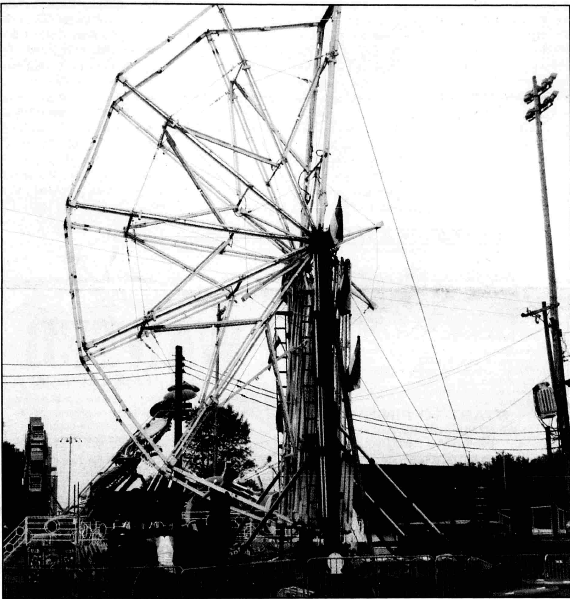
A ferris wheel in the process of being erected last weekend is now in full swing for the fair.
