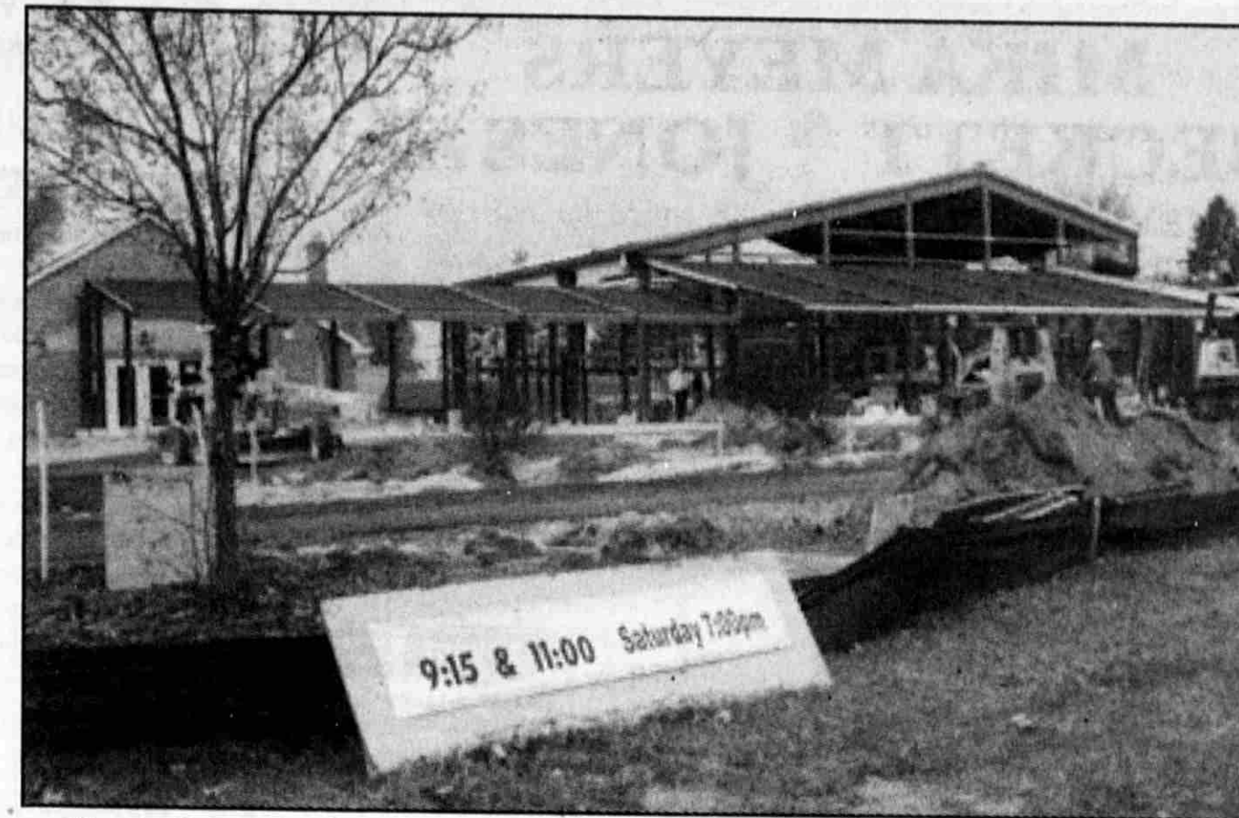
Sign in front of Impact Church shows services continue during construction.
