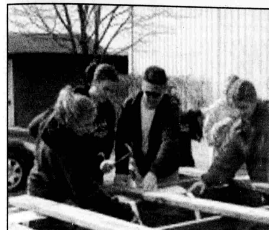
Sections of floating dock were hammered together.
