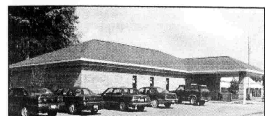
What started out as a frame on Wednesday was a fully constructed Jehovah Witness Kingdom Hall by the end of the day on Sunday.
