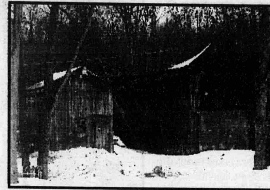
A heavy December snow causes the roof of a barn owned by the Towers family in Fallsburg Historical Village to collapse. O.E. Bieri is hired to take down the entire barn with instructions to save the siding to be reused when a replica is created.
