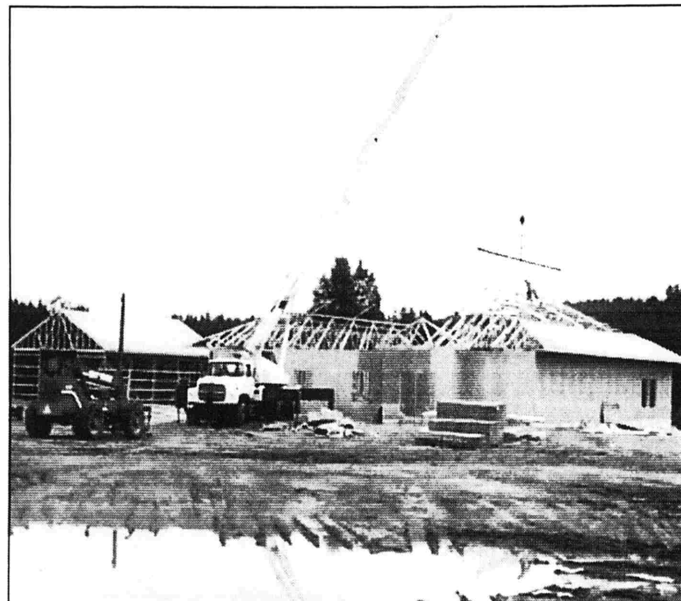
Construction crews finished framing in the Wittenbach Agri-science Center.
