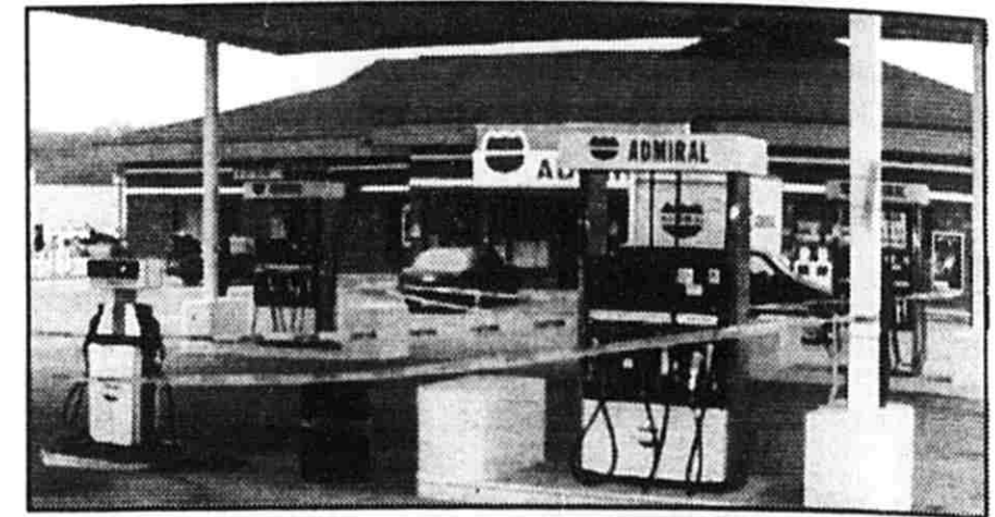
Lowell Area Fire Department doused the flames of a fire in the northwest room of the Admiral station, preventing any significant structural damage.
