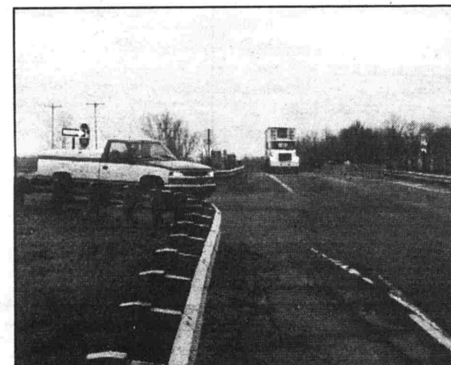
A multi-way stop is put in at the M-50/I-96 overpass.
