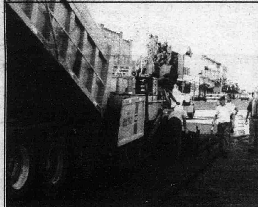
The M-21/Hudson Street intersection was shut down for roughly 15 hours on Saturday while crews laid a new water main and then repaved the intersection.
