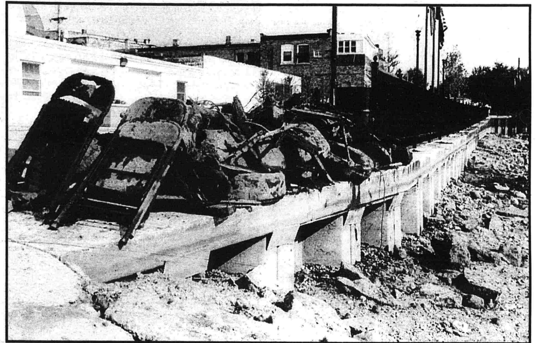
Pipes, tires, rims, a refrigerator and many miscellaneous items were found on the bottom of the Flat River during a cleanup project.
