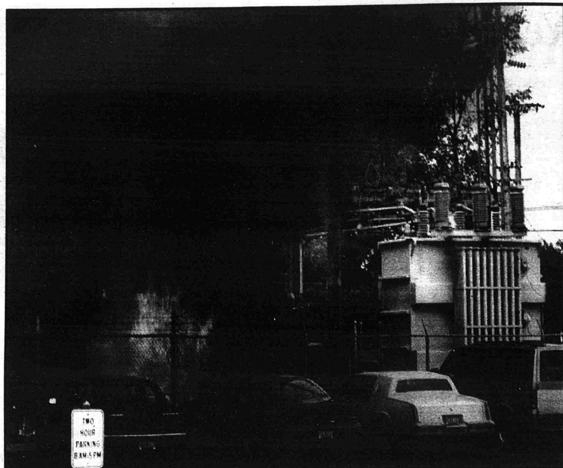
A transformer explosion at Lowell Light & Power leaves 2,100 customers without electricity.
