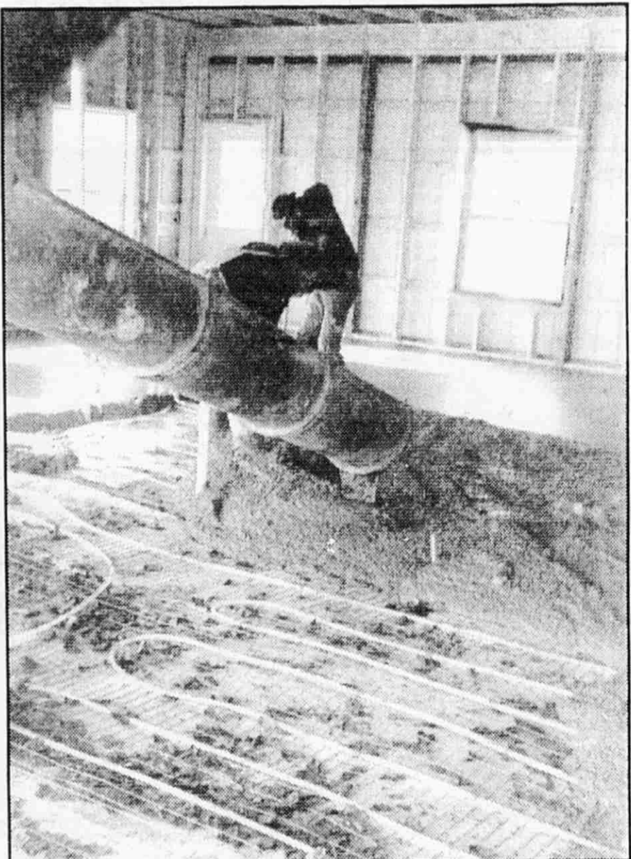
Contractors work to pour the cement floor at Arctic's new building.
