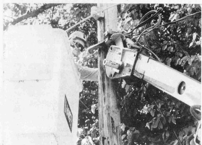
Power and telephone lines had to be taken down and put back up so that the 75-tor house could be moved.
