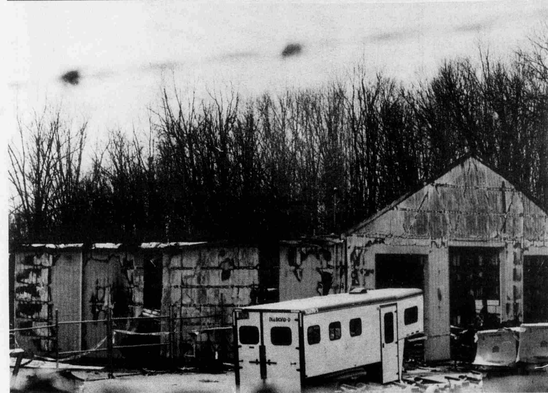
A Saturday morning fire turned Rockford Marine's warehouse into hot ashes. There was an estimated $500,000 worth of damage.
