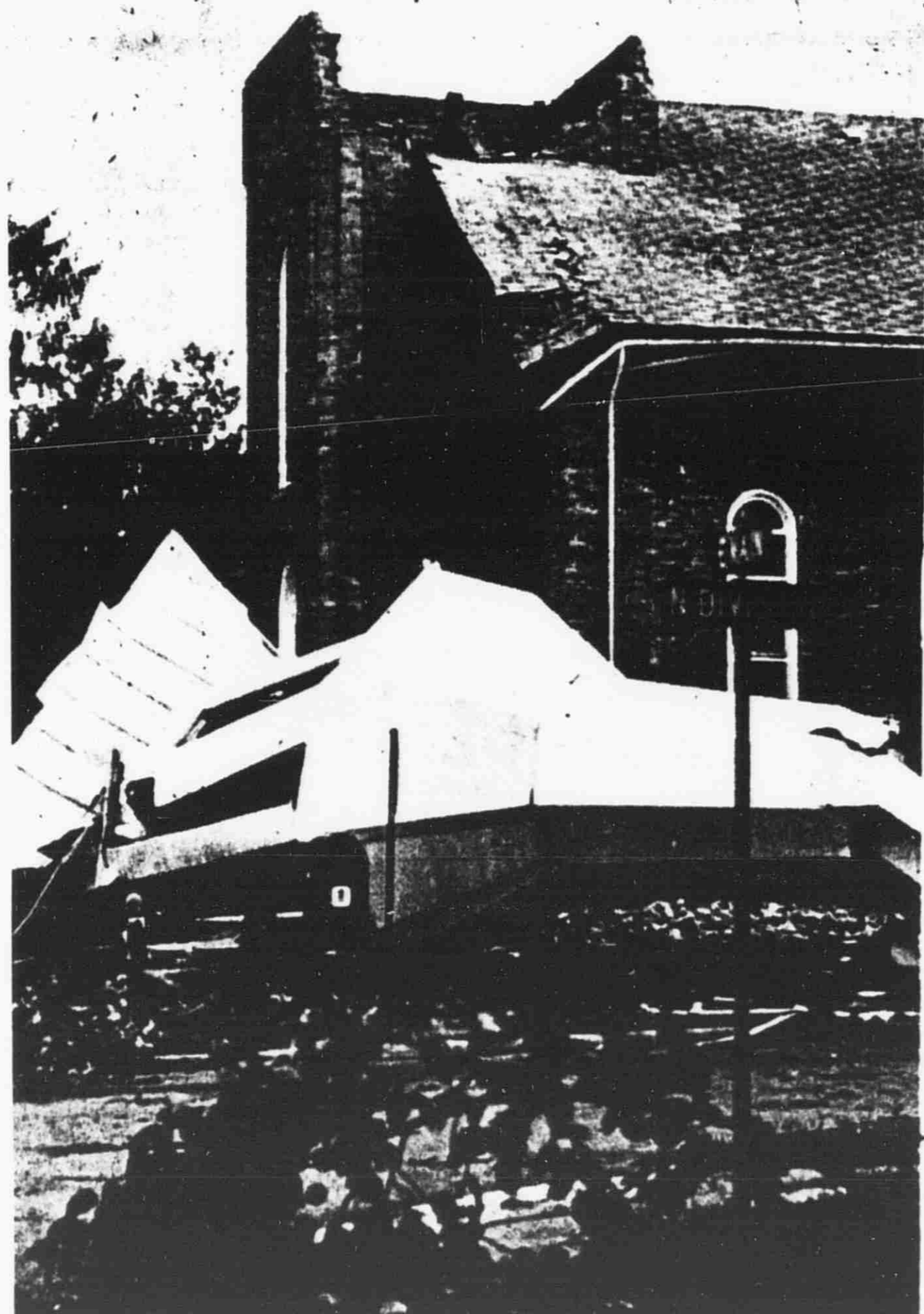
Ripping the steeple off from the First United Methodist Church of Lowell was one of the most sensational bits of destruction that the wind dealt out. The belfry portion of the steeple is more than 100 years old, but the very top section of the structure was erected in 1967.
