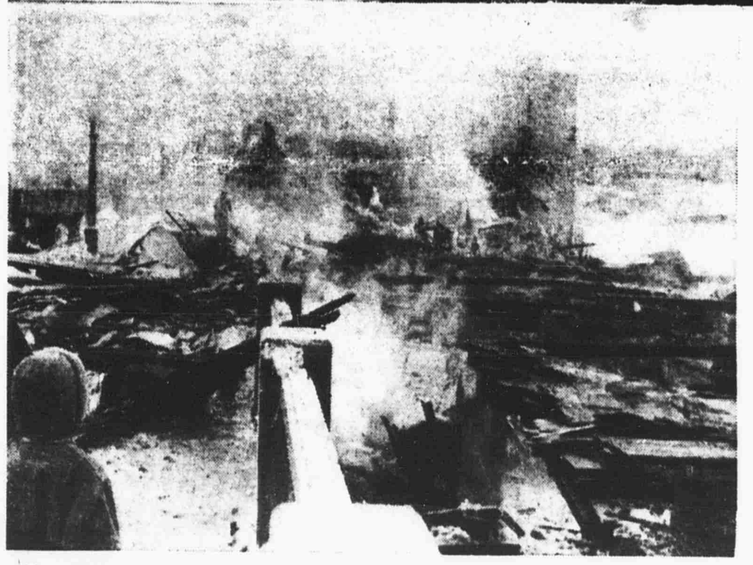
Top view is a picture taken shortly after 7:00 a. m. on Thursday morning, January 2 showing the big start the fire had before the fire department arrived. Flames roared into the sky lighting up the entire area. Light poles forty feet from the buildings caught fire and had to be extinguished by utility plant line superintendent, John Jones. The second view is one of the firemen concentrating their entire supply of water on the
