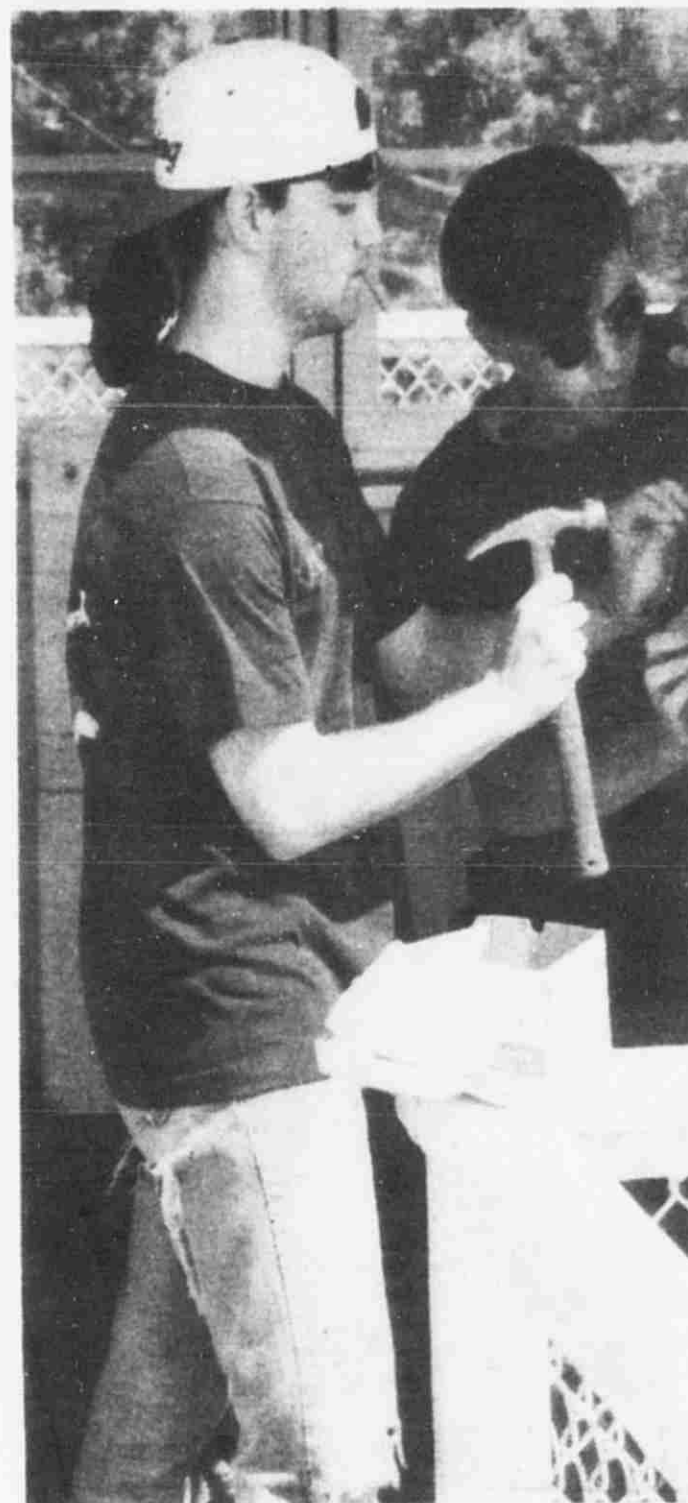
Brandon Triplett and Jason Myers repair a door frame.
