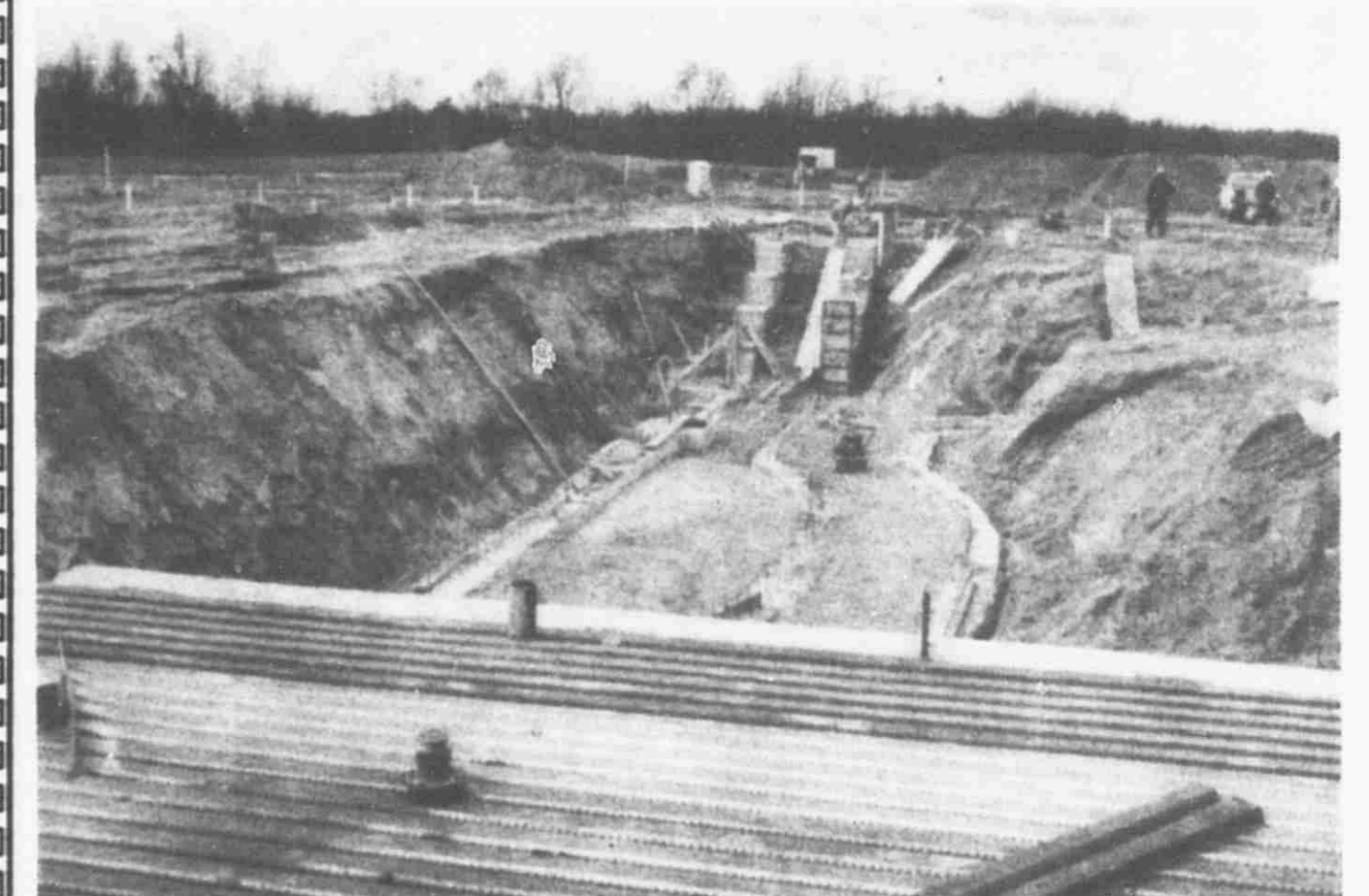
The foundation for the orchestra pit has been dug out.
