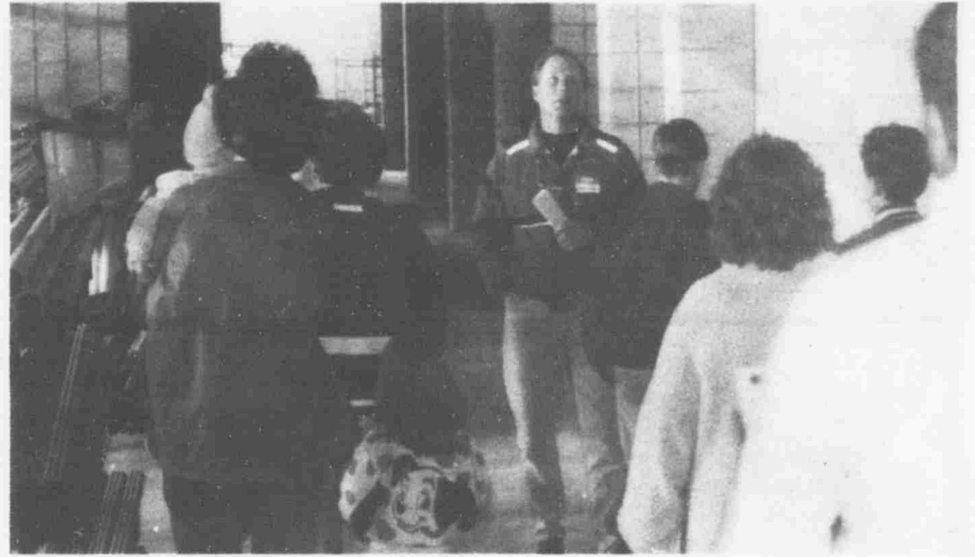
Scott Vashaw walks one of 16 groups through a portion of the new high school that is now under construction.
