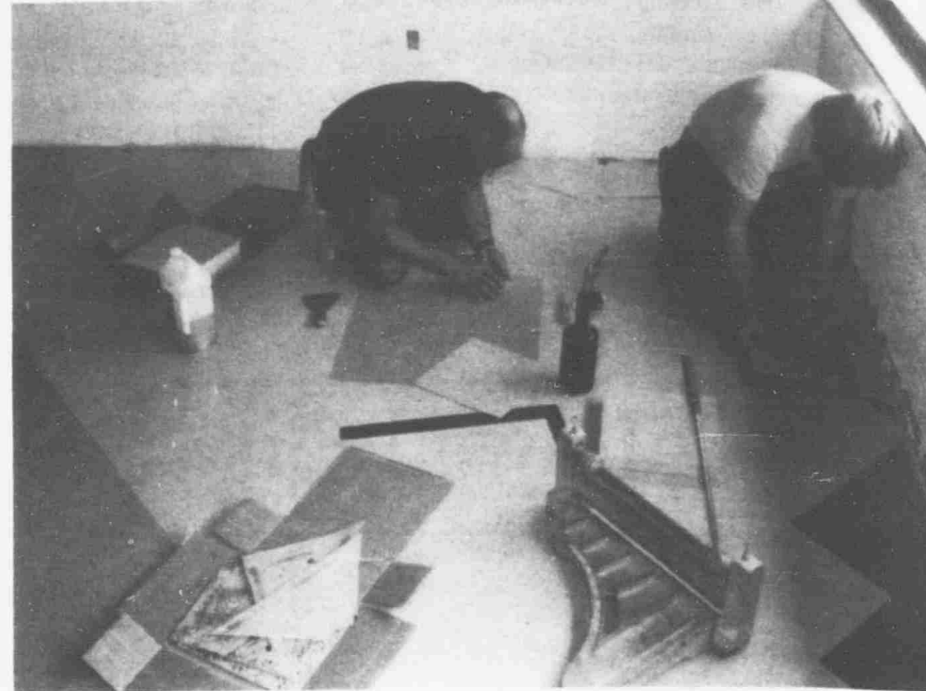
Tiling an Alto Elementary floor.
