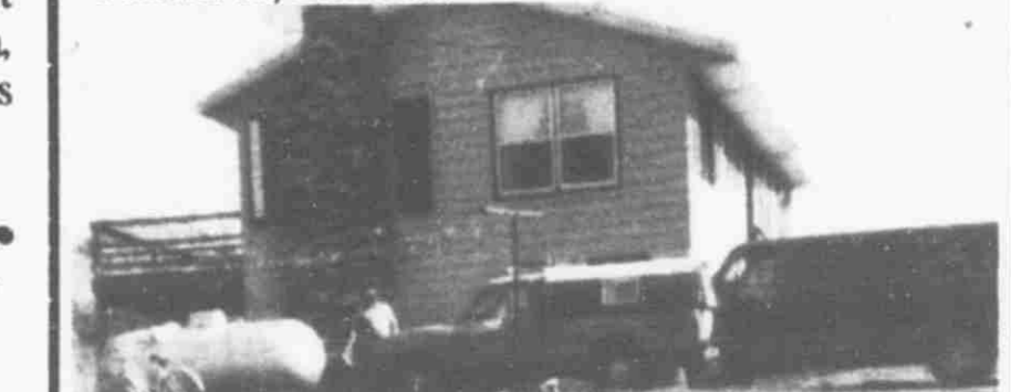
3 BEDROOM - 14 year old home, only 2 miles west of Saranac. Has 2 fireplaces, 1 1/2 baths, full walk-out, basement, 2 1/2 acres, $62,500. Call Art Schmidt Jr., 363-9875.
