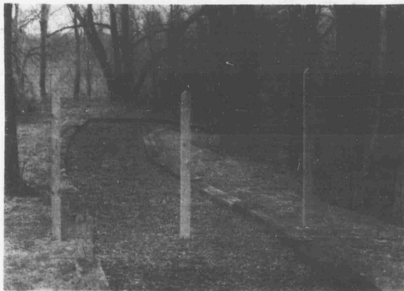
The walkway leading down to a new canoe landing on the Flat River is a gentle grade covered with shredded bark. Posts have been erected to keep motor vehicles out.
