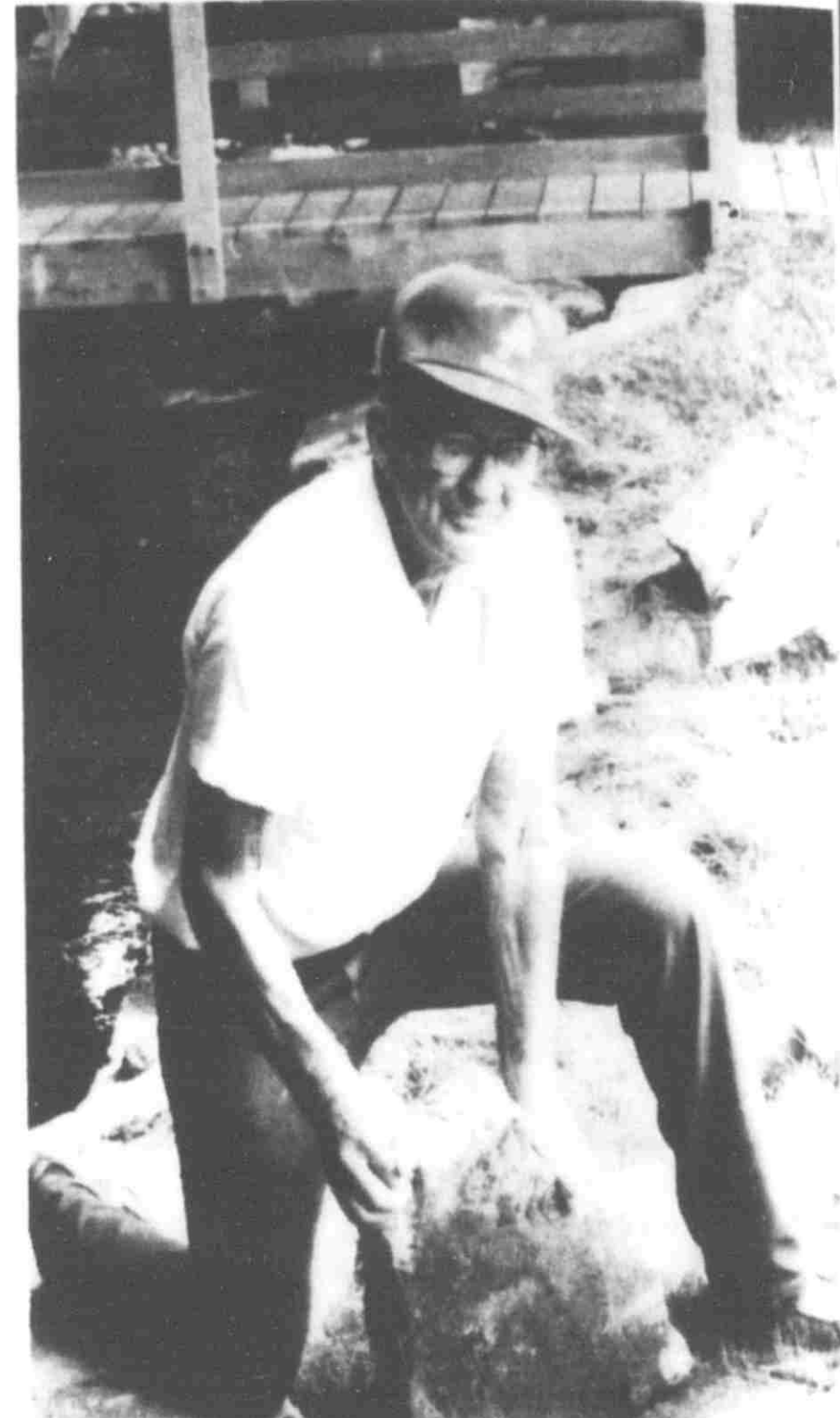
Sam "Babe" Wingeier finishes up some landscaping work around the bridge.
