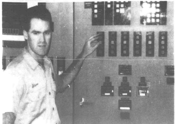
This panel controls the sequence at which the wheat tempering bins fill and empty.
