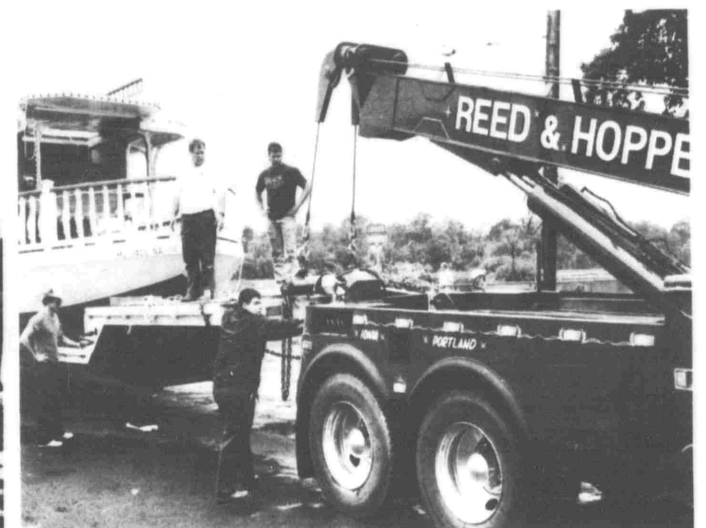
Lowering the "Princess Laura" into the water was quite the chore.
