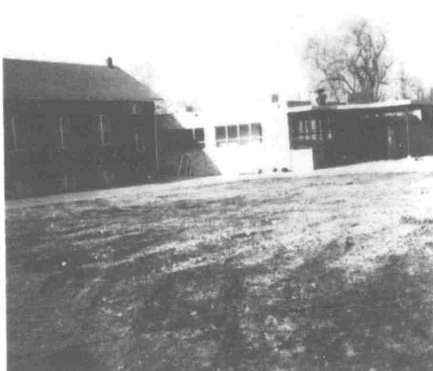
The "connector building" at the First United Methodist Church will be Consecrated in a special service on Sunday, May 13.
