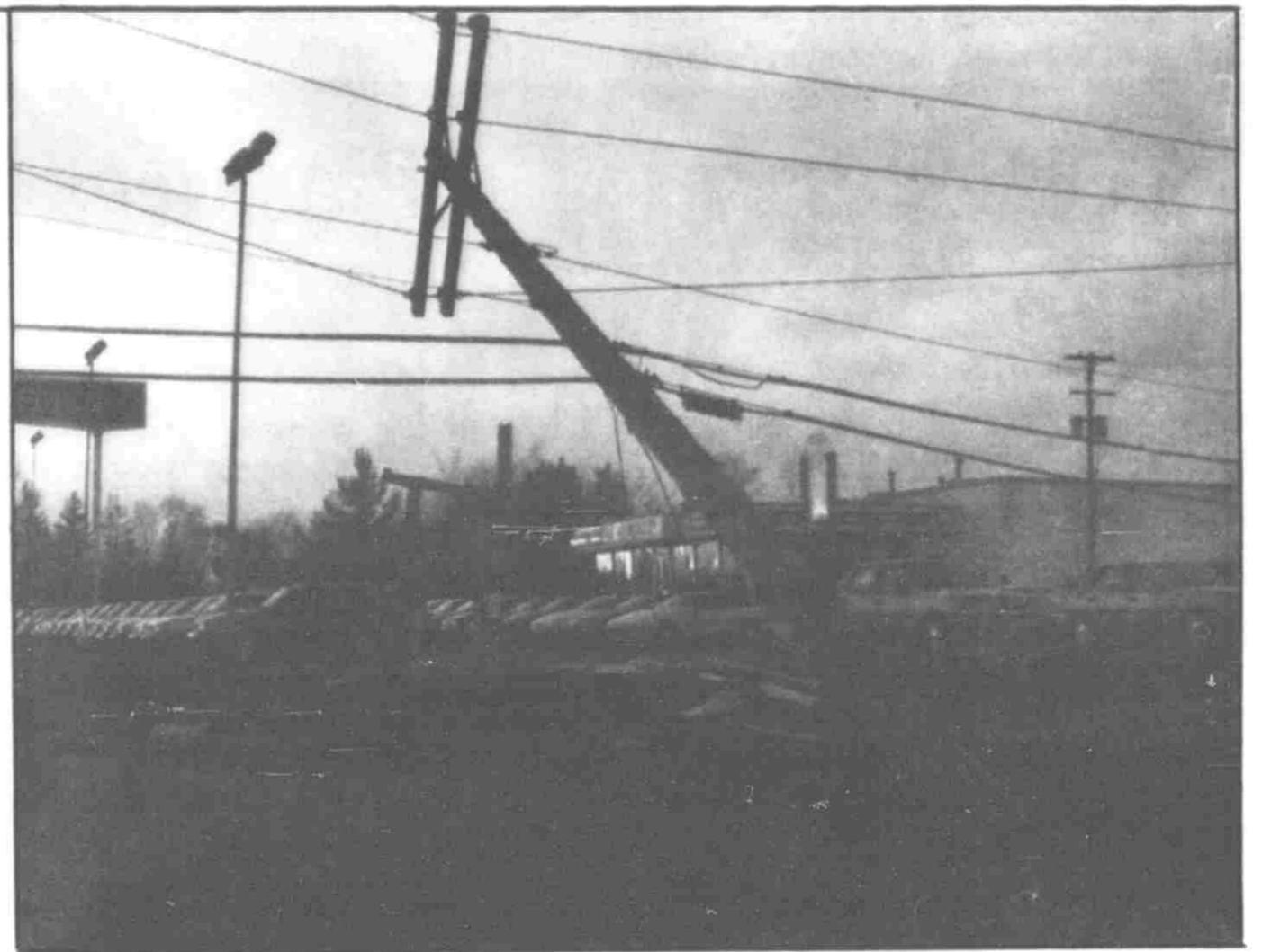
The electrical pole was broken in three different places.
