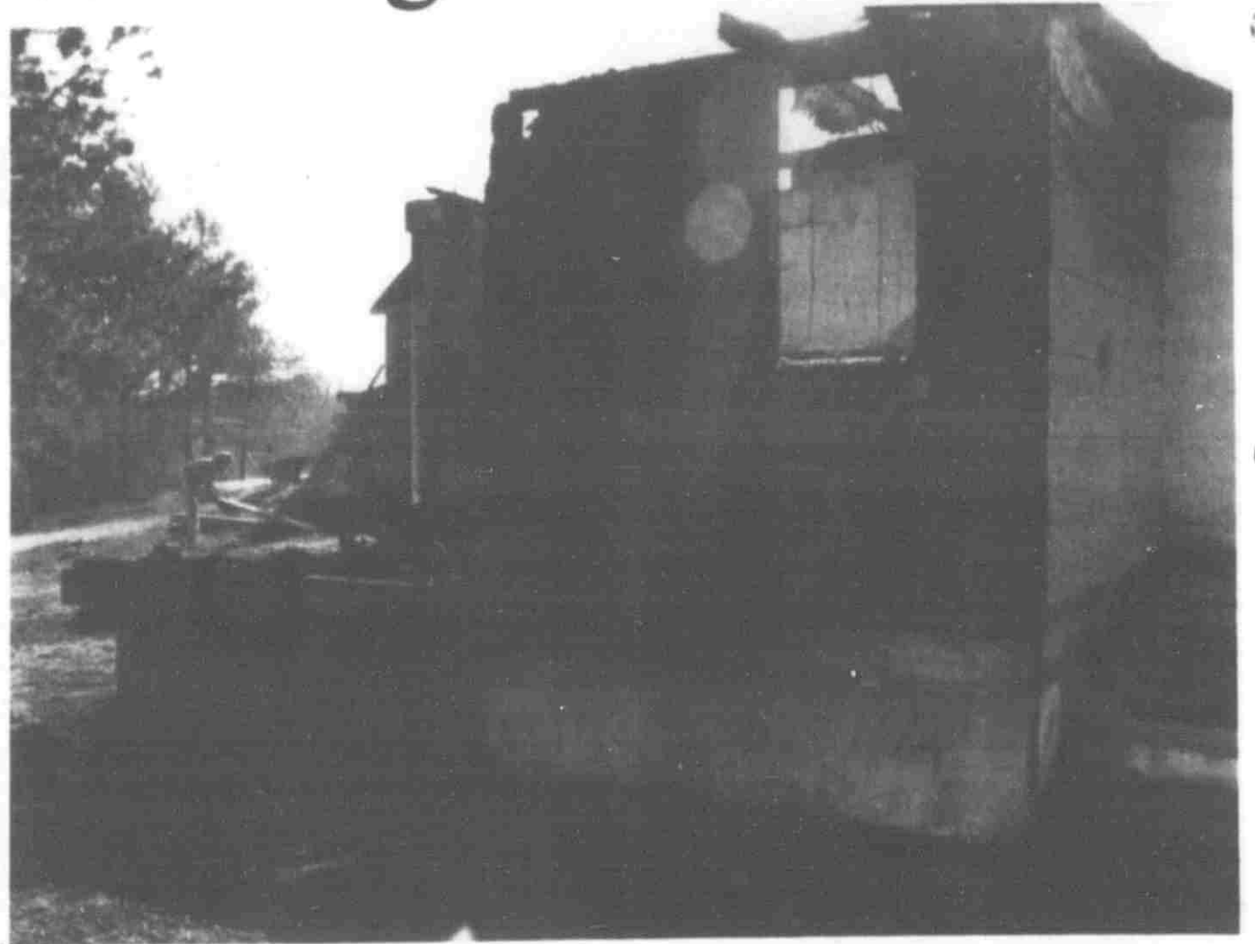
A Wednesday night fire was responsible for $10-$12,000 worth of damage at the Stephanie Hilton home at 2580 Lowell View Dr.
