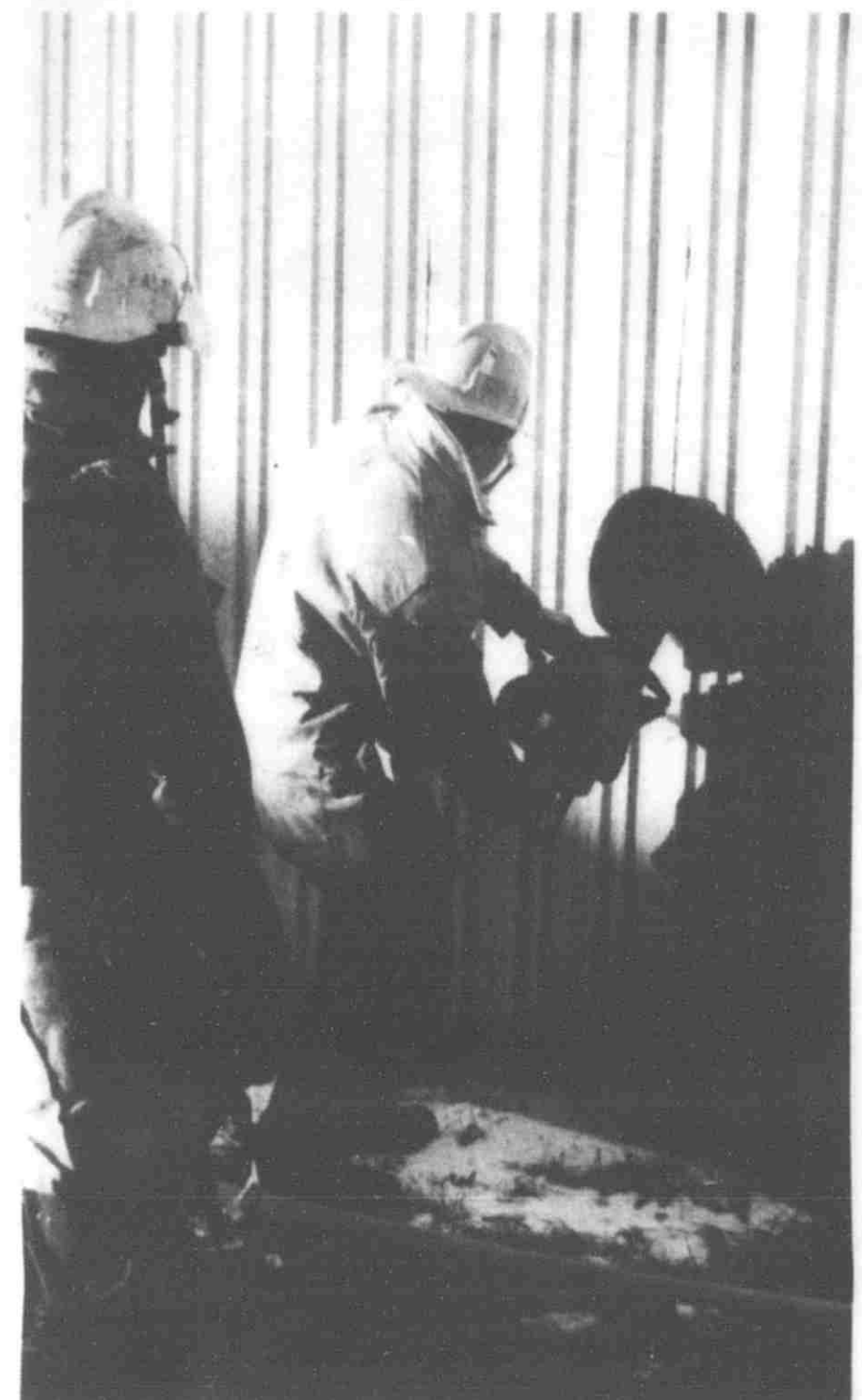
An electrical box on an inside wall was the cause of the fire, according to Alto Fire Chief Jerry Posthumus.
