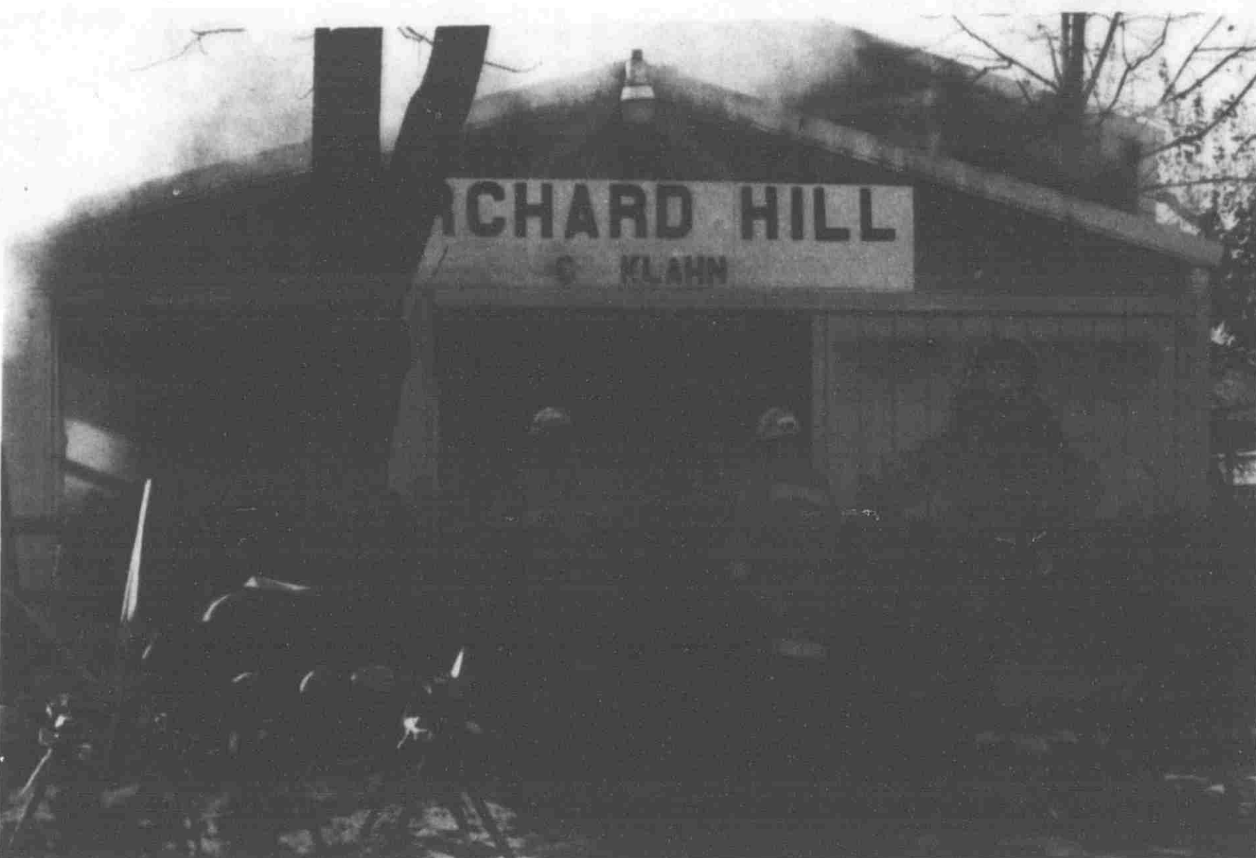
Klahn's Orchard Hill Farm storage building burned in a Dec. 8 morning fire.
