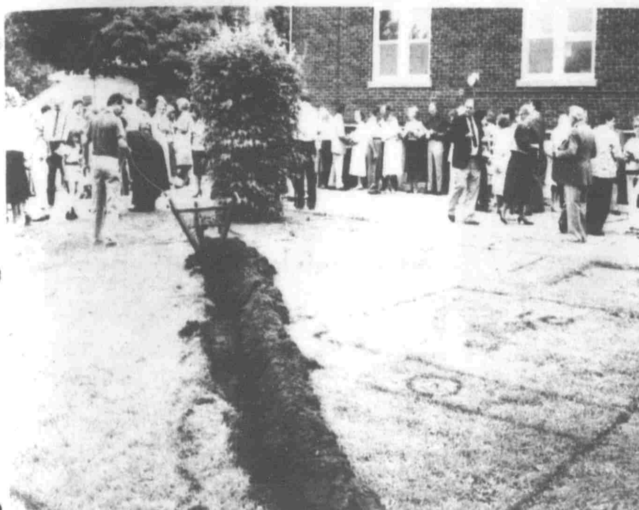
Members and friends of the First United Methodist Church all had a hand in the ground-breaking ceremony.
