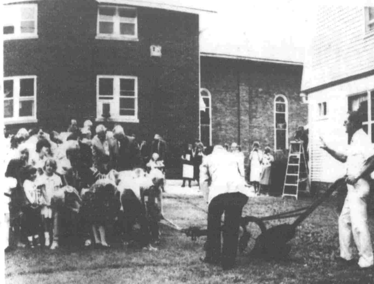
Ground was broken for a new connector building Sunday, July 30 at Lowell's First United Methodist Church. The commonly used shovel was disregarded. Used in its place was a one-bottom horse drawn plow owned by Arie and Ruby Leeman.
