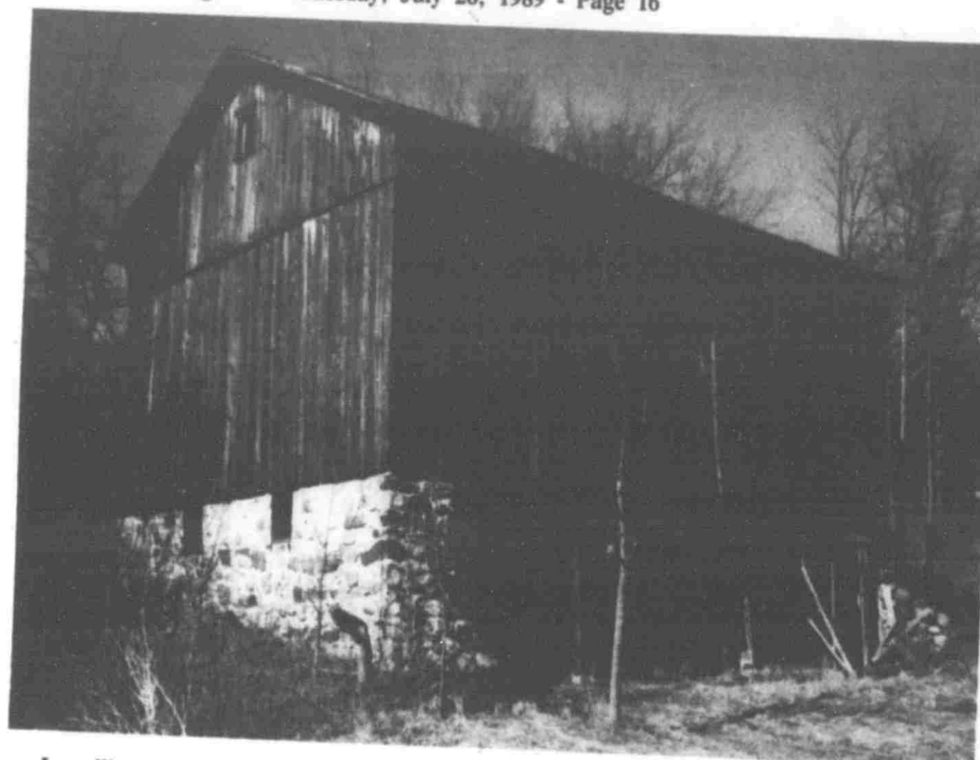
Lowell's West Central Michigan Historical Society is busy with its restoration of the John Wesley Fallas barn.
