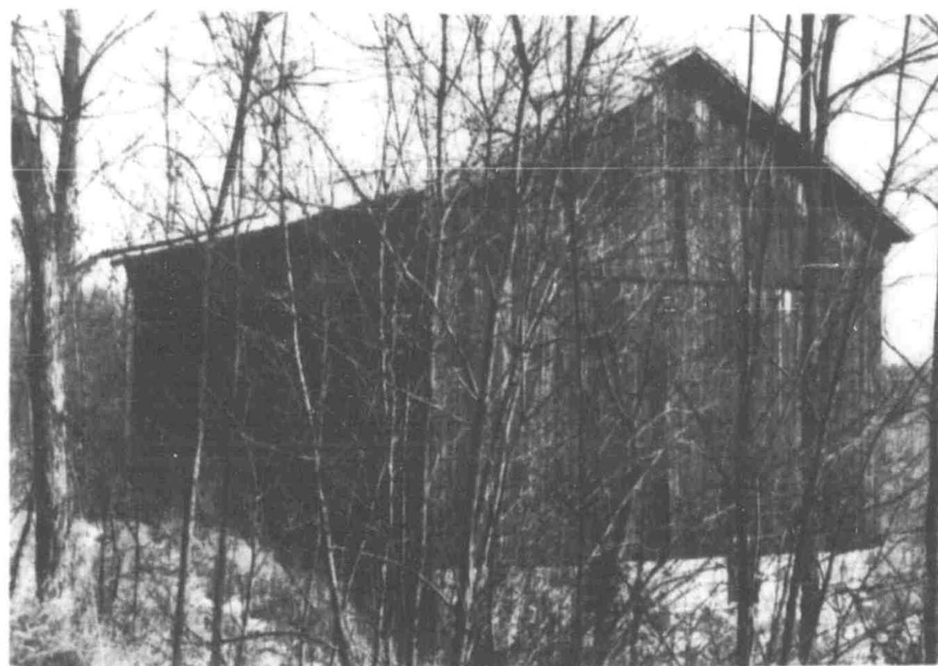
The second building which the historical society will purchase is this barn which was built in 1896 by J.W. Fallass' sons.
