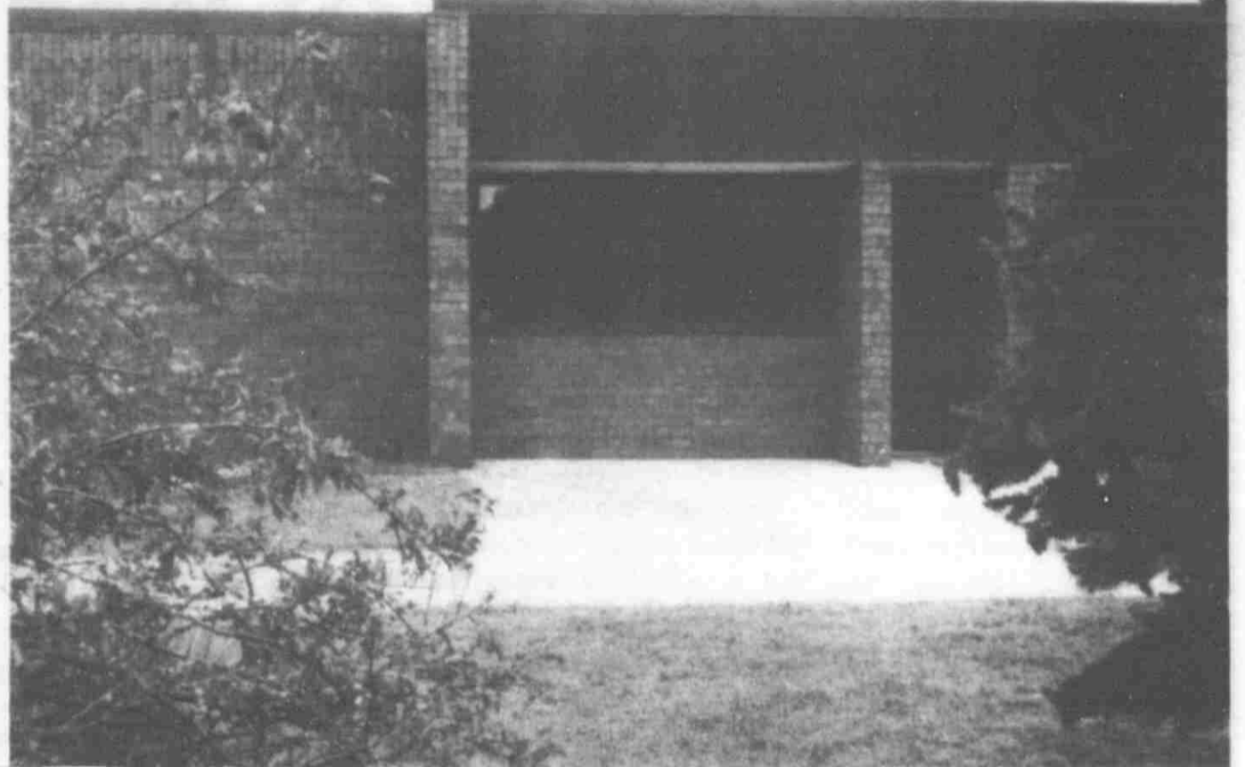
The art and graphics room on the northeast end of the Lowell Middle School will be used by the senior neighbors. This door will provide the seniors an entrance and exit to and from their room.
