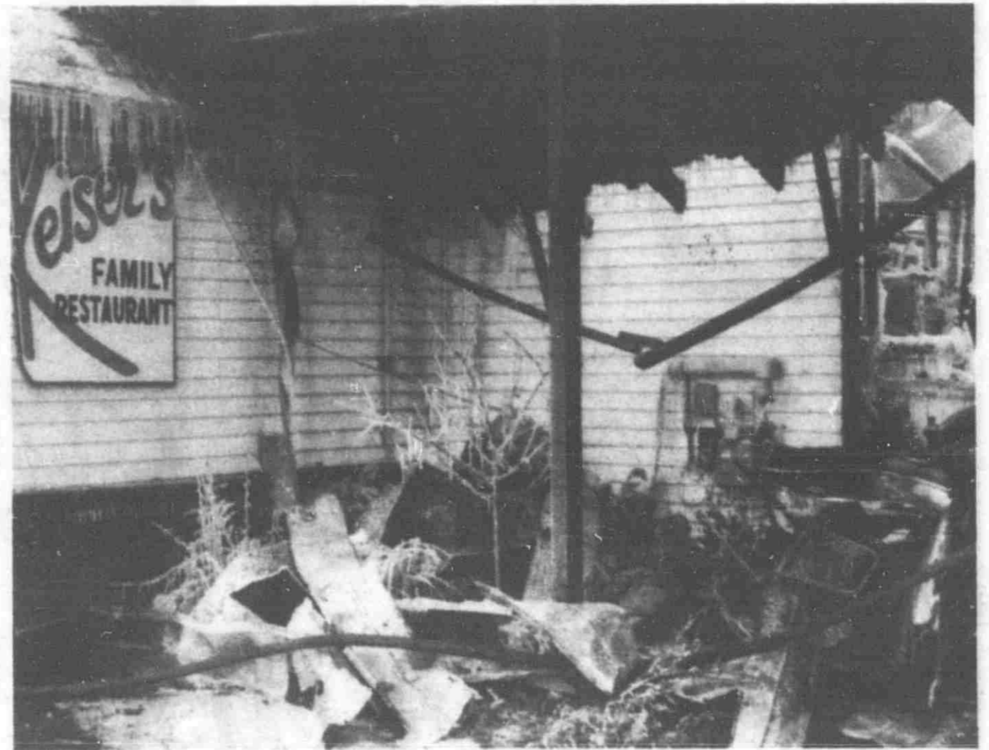
The morning after, showed the aftermath, of a fire that destroyed the building of Lowell's oldest merchant. The state fire marshal report stated that the cause of the blaze at Keiser's Kitchen was electrical.
