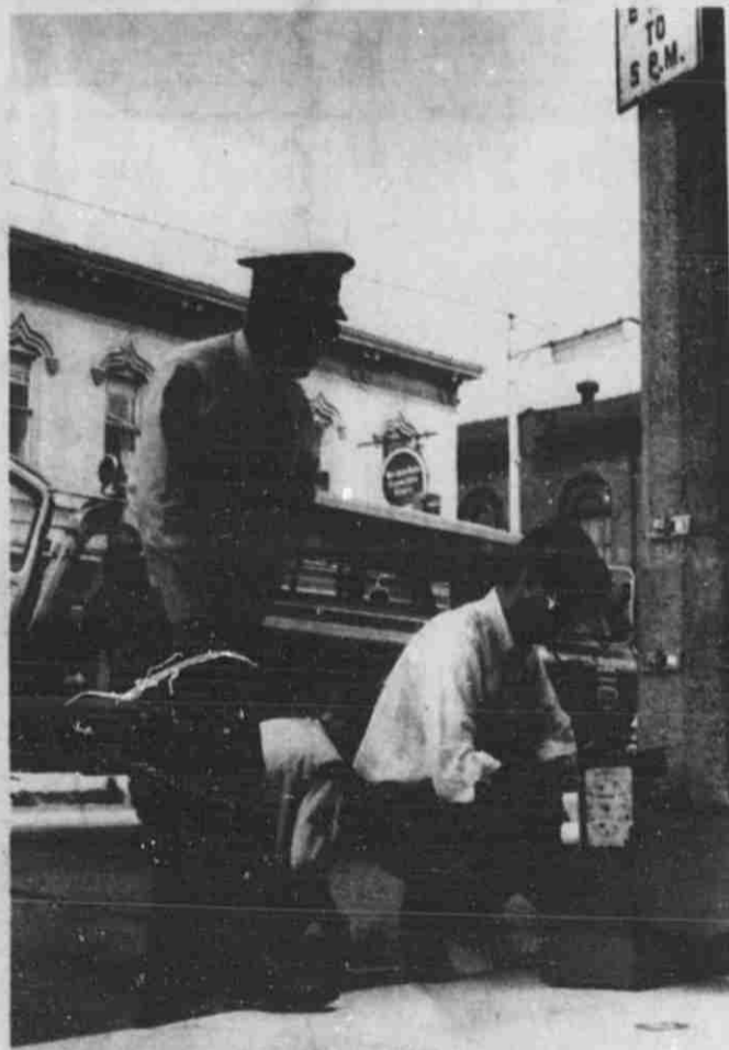
TRAFFIC STOPPER? Lowell Police Chief Avery Block looks on as members of the Michigan Highway Department install traffic-counters near the intersection of Main and Monroe as part of a survey to determine the need for a stop signal at the busy intersection. Results of the survey are expected to be known in a few weeks.
