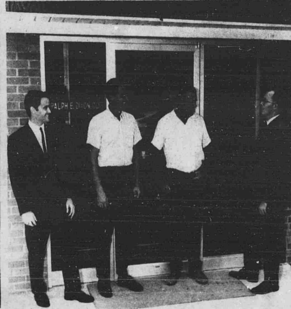
NEW PROFESSIONAL building opened in Cascade with Dr. Ralph E. Nixon, DDS (left) greeted by Irving and Everett Marsman, and Dr. Stephen K. Marsh, MD (right) builders and owners. —Photo by Scott Jefferies
