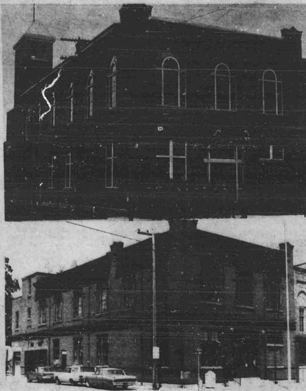
NOT TOO MUCH has changed as far as Lowell's City Hall is concerned. The picture above shows how it looked in the old days . . . and the one below as it appears today. The bell tower and potted plants have disappeared, but most everything else looks the same.
