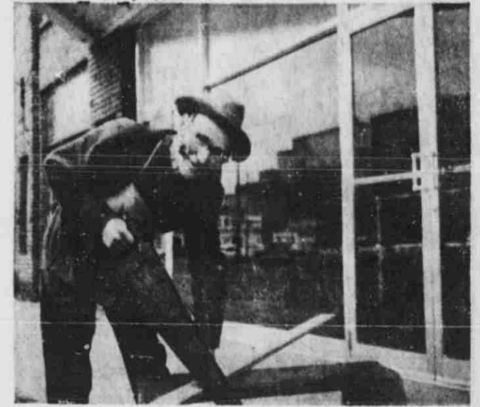
Earl Evans, owner of Strand Theatre, 315 W. Main Street, is pictured above hard at work on the renovation of his theatre. Owner-operator of the theatre for the past eighteen years, Evans is enthusiastic about his plans for the future of his business.
