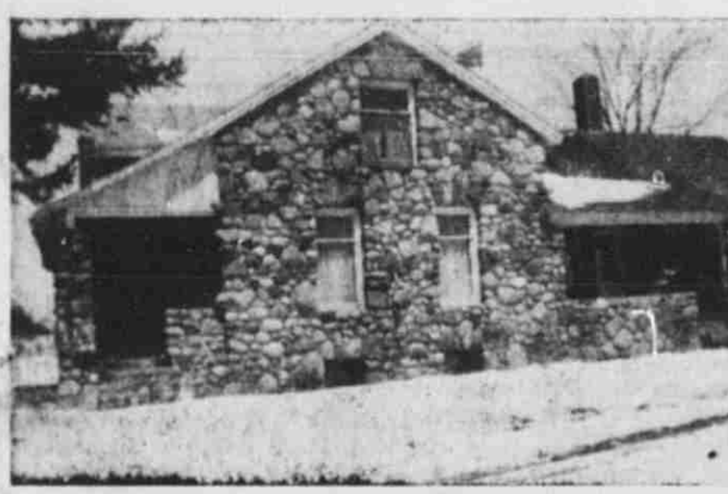
Pictured above is the home of Mr. and Mrs. C. O. Condon, newly designated a centennial farm. The frame house was converted to cobblestone about thirty-five years ago by C. O. and Laura. It is a very outstanding house on Fallsburg Park Drive and many people stop to take pictures, while out Sunday driving.
