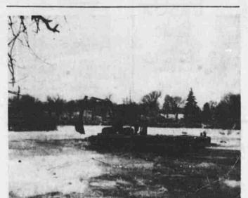
Somerville Construction Co. launched a barge on the Flat River near the Junior High School this week and began digging a trench in the river bottom for a new high pressure gas main. This main will give the west side of town an additional feeder in case of a break in the Main Street line and also take care of the needs of the Light and Power plant's new gas-burning generating unit. The trench the gas main is laid into is four feet below the river bottom.
