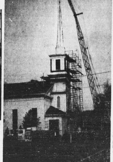
A new, 30-foot steeple for the Lowell Congregational Church was lifted into place by a crane in October, replacing the building's original steeple, which had been torn down in 1925 after it had been damaged by high winds.
