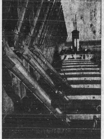
Londing iron ore at an upper peninsula port is one of the more than 300 Great Lakes ships which represent the vital transportation link between iron mines and the nation's blast furnaces. These boats, traveling the Lakes from spring to winter, have carried an average of more than 78,000,000 tens of iron annually since 1940. Michigan ranks among the nation's leading iron ore and steel producers each year.
