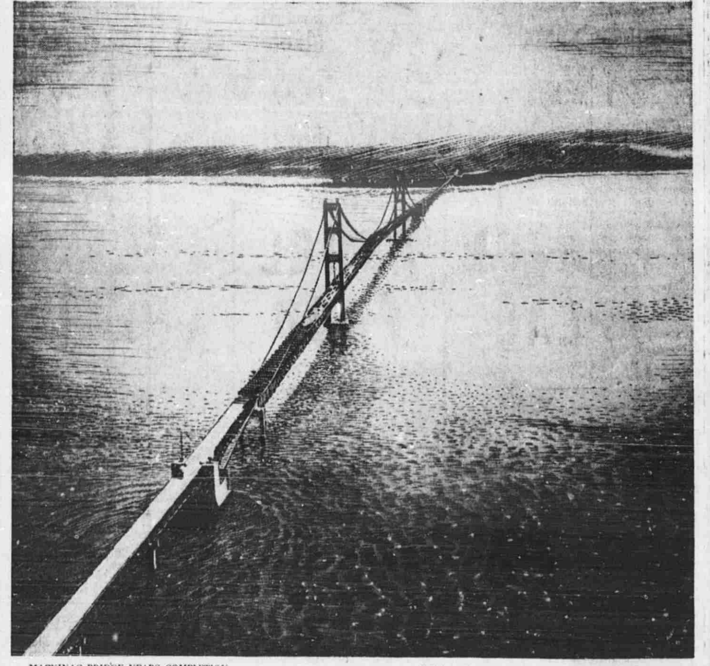
MACINAC BRIDGE NEARS COMPLETION. Full Color Reproduction suitable for framing sent upon request.
