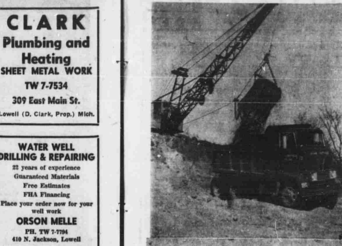
No Hold-up On Bridge Construction
