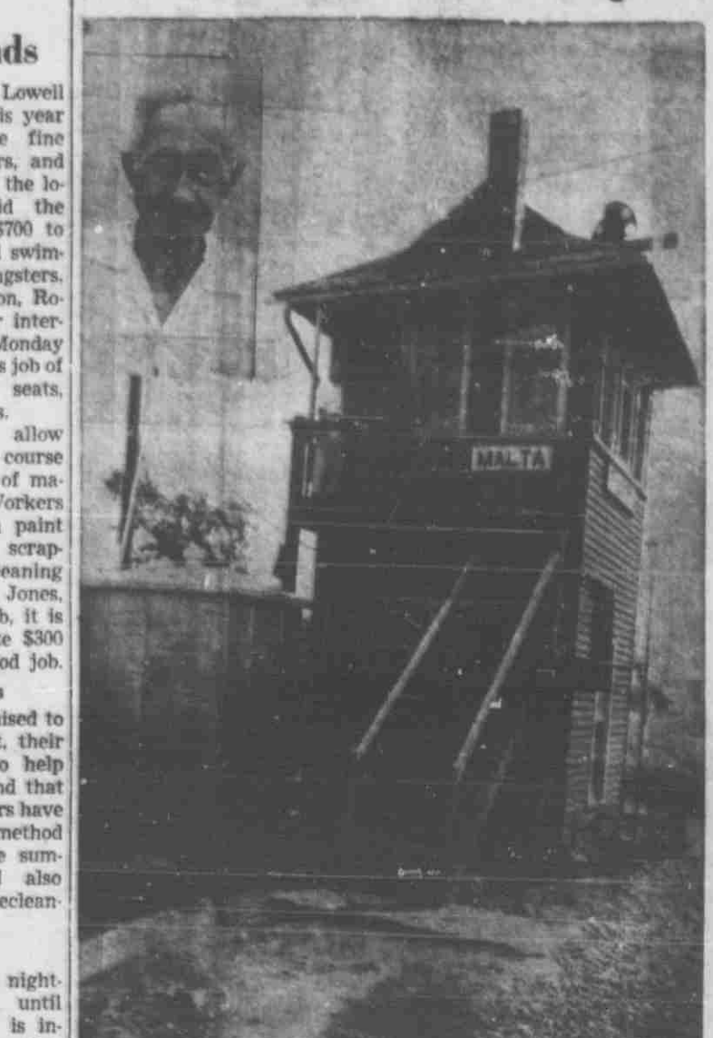
With over 50 years of service keeping trains on the Grand Trunk Railroad and the Chesapeake and Ohio from meeting at the track crossing, Malta Tower, located in Segwun, gave way to progress last Monday at four p. m. when a new "automatic interlocking plant" (left) took over the duties of the five operators who manned the tower on an around-the-clock basis. M. R. Wood (insert picture) was the last full time operator to be stationed at the tower.
