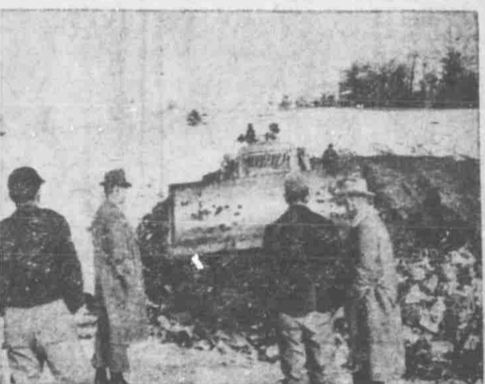
Residents of Boston Township gather for the state inspection of Lowell's sanitary land fill. Tom Moore (right), Lowell's Supervisor of Public Works explains the bulldozing operation to members of the group, showing that all refuse collected will be covered and packed with dirt, leaving the area neat and odorless.
