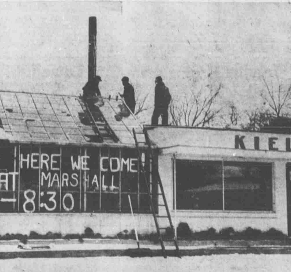
HERE WE COME! A hail stone about the size of a baseball hit the glass in Kiehl's Greenhouses on Friday night's storm. The Kiehl was away at the time and is truly thankful that Lyle Covart and son Bill, along with Elmer Laver realized the great amount of damage that could be done to the glass panes and covered the holes in the roof with canvas and heavy paper to keep out snow and cold.
