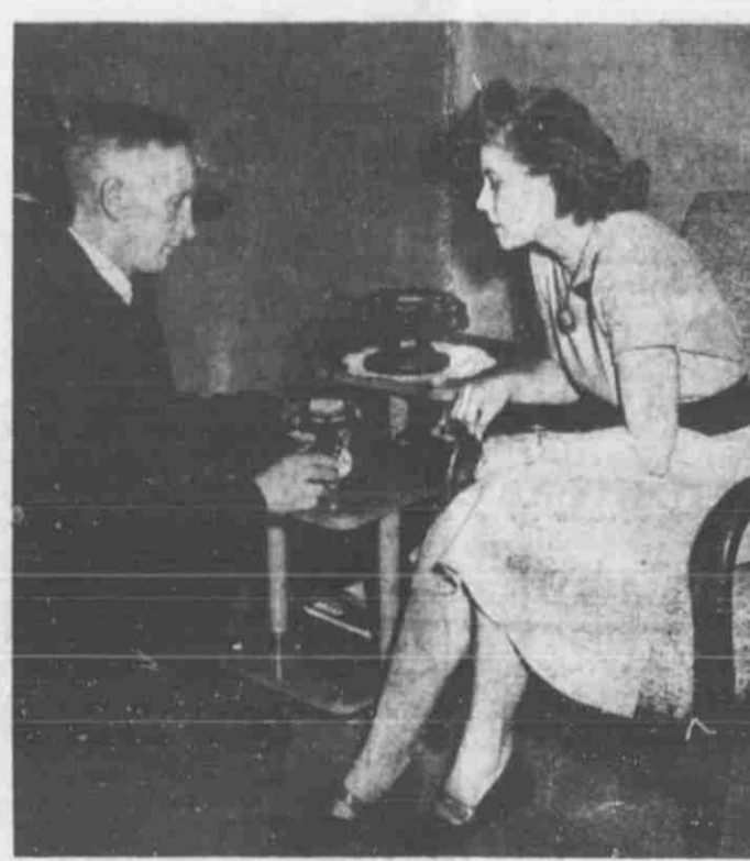
Mrs. Richard Schleritzauer looks on as Wayne "Whitey" Schroder, veteran Michigan Bell Telephone Company employee, installs a dial telephone instrument in her home in preparation for the changeover to dial operation here on January 8.
