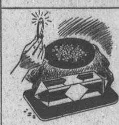
ONE UP ON NATURE-During the war Bell Laboratories scientists found a way to grow synthetic crystals better in some ways than natural quartz. A "seed" crystal is produced by evaporating chemical salts, then rotated in a chemical solution which causes deposits to build it up to many times its original size. Crystals vibrate at exact frequencies, separate the many telephone messages traveling over a long distance line.
