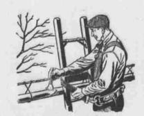
**BLOWING BUBBLES** - To help keep telephone service reliable, thousands of miles of Long Distance cables are filled with harmless nitrogen gas. If a cable is damaged, the gas pressure drops and sets off an alarm indicating the pproximate location of the damage. To find the ctual break in the cable sheath, if it's so small can't be seen, the repairman may paint the cable with soapsuds - the exact point of damage being indicated by bubbles blown by the escaping gas.
