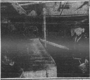
Farm labor specialists of the Michigan State college extension service suggest this "cafeteria" system of feeding ground grain on the spot. Clyde Partridge, of Rockford, installed his semi-automatic grinder in the feed alley of the dairy barn to save steps and labor. A small hammers is mounted on a tall dust-tight box, and whole grain mixtures are fed by a chute from a bin above which is large enough to hold a week's supply.
